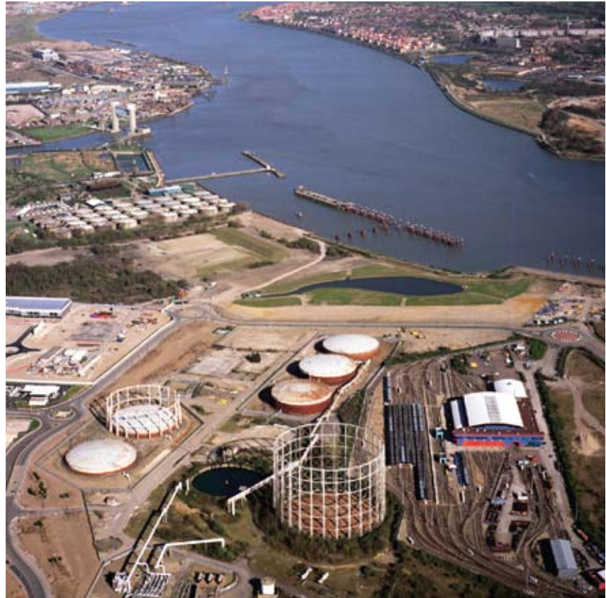
National Grid Property is set to make cost savings on work at the Beckton Gas Works site as a direct result of involvement with NISP
